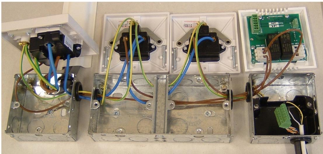
In the UK the wiring should be done in accordance with the 16<sup>th</sup> Edition Wiring Regulations and to comply with Part P of the building regulations. An appropriate inspection or certified installer should be sought.
