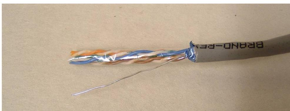
Unwrap the outer clear plastic sheath which covers the 4 twisted pair cables and drain wire and remove this.
