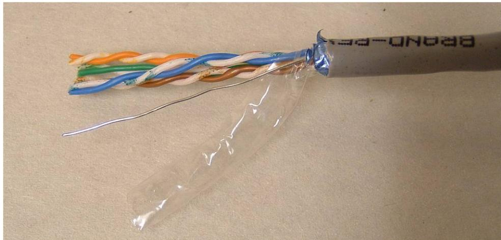
Separate the 4 twisted pairs (still keeping them loosely twisted) and place the brown pair aside, as this is not normally used (if this is to be used to double up ignore this stage). Strip the end of the wires using suitable wire strippers being careful not to nick the copper core, as this will make it liable to fracture if flexed.
