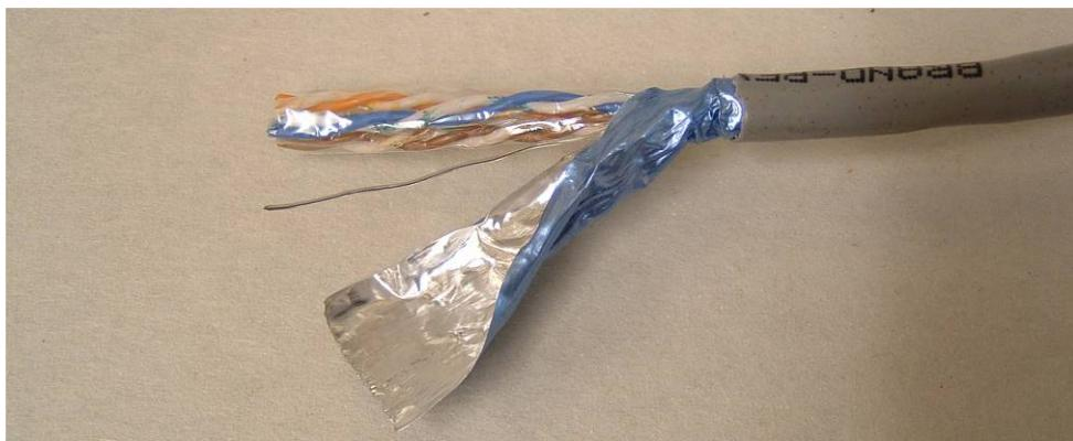
Peel back the screen to reveal drain wire and inner cores. Cut or tear away the foil screen being careful not to damage the bare screen drain wire.
