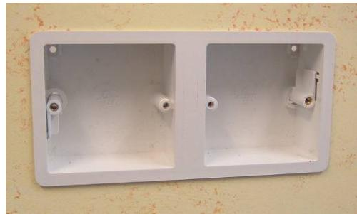
Note: No rotational adjustment is provided by the DFP mounting bracket. The Pattress should be fitted as level as possible. Some metal pattresses allow level adjustment. The left hand side is used for the low voltage wiring to the Cat5 cable for the IDRANet network signals. The right hand side is used for switching mains voltage.
